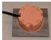
Insert the whole thing in the opening and screw the wooden cover down with both 3 x 20 Spax screws.
